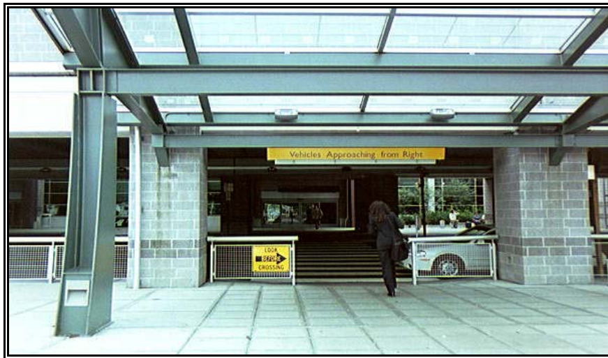
Lower Level Terminal Crosswalk
